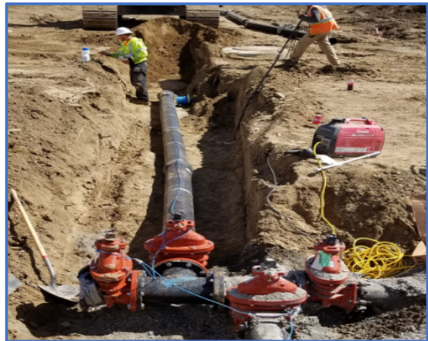
Photograph of District job site, including valves
