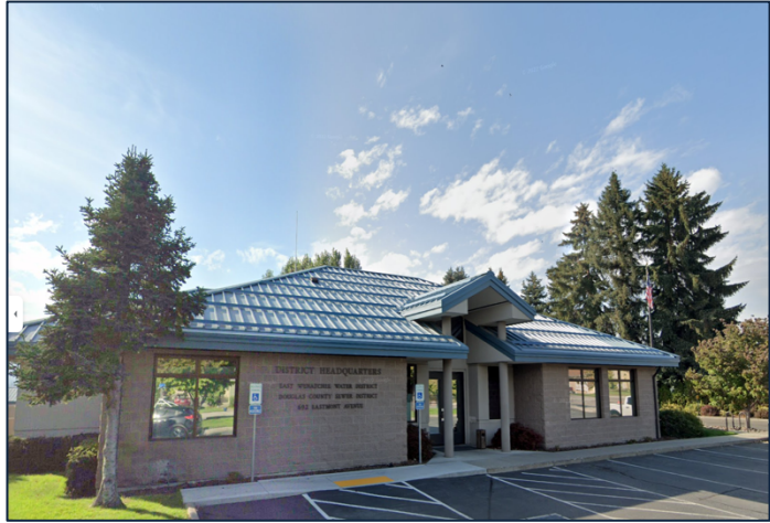
Water District Headquarters, East Wenatchee, Washington.
